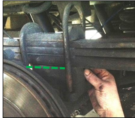
Removal of U bolts
